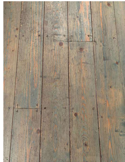
Photo 47 - Treated floorboards
