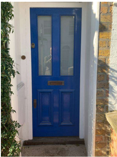
Photo 26 - Main front door
