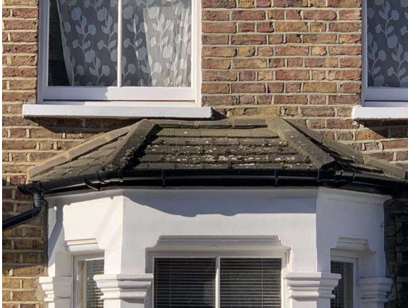
Photo 4 - Roof over bay window
