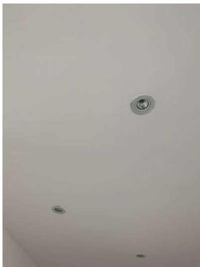
Photo 38 - First floor landing
