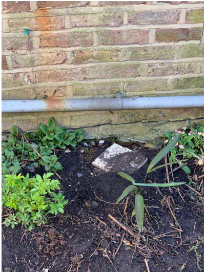
Photo 18 - Visible damp proof course to new rear addition.
