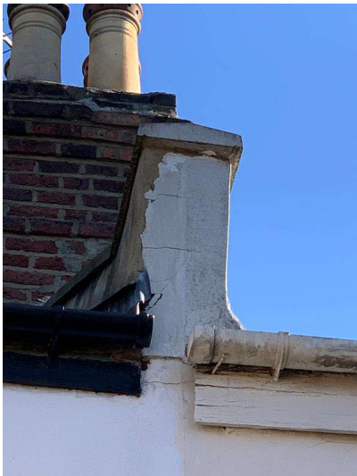
Photo 8 - Parapet wall: Rear left
