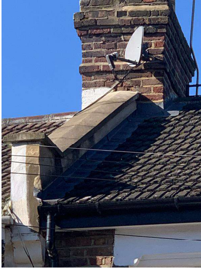
Photo 6 - Parapet wall: left hand side
