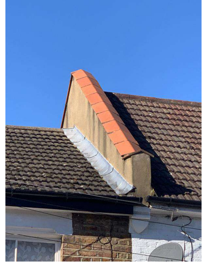
Photo 7 - Parapet wall: Right hand side
