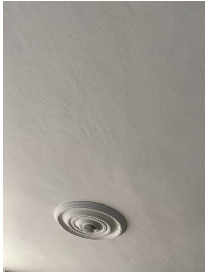
Photo 36 - Living room: lath and plaster
