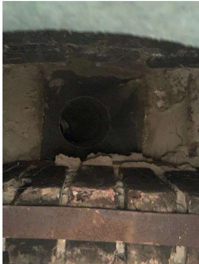
Photo 62 - Lined chimney flue
