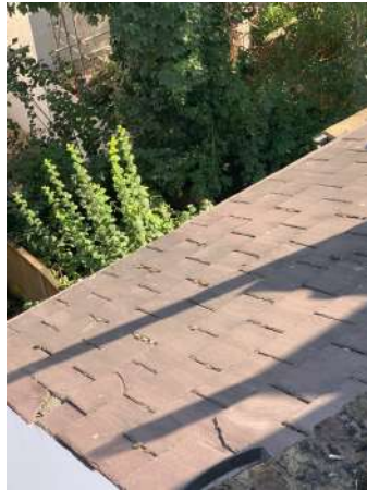
Photo 3 - Rear addition roof
