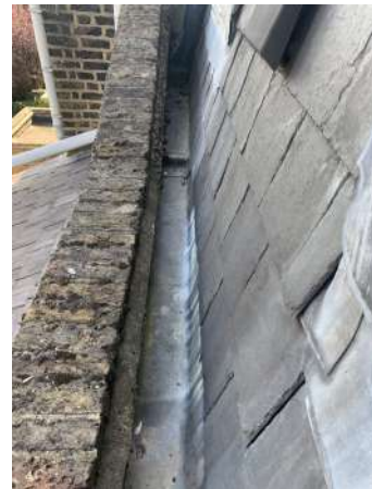
Photo 11 - Box gutter
