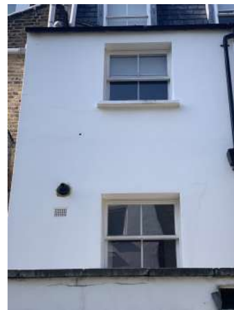
Photo 22 - Rear wall to rear addition
