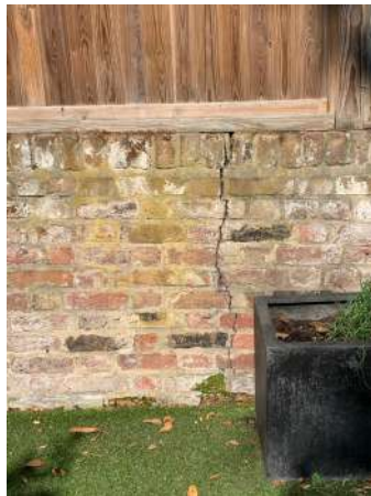
Photo 33 - Cracked brickwprk
