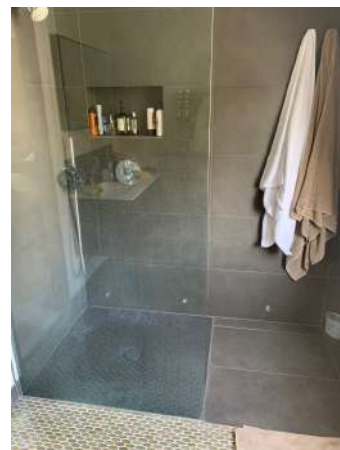
Photo 59 - 3rd Floor shower room
