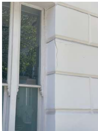
Photo 15 - Cracked render
