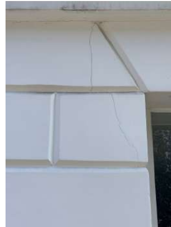
Photo 14 - Cracked render
