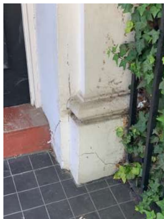
Photo 17 - Cracked render
