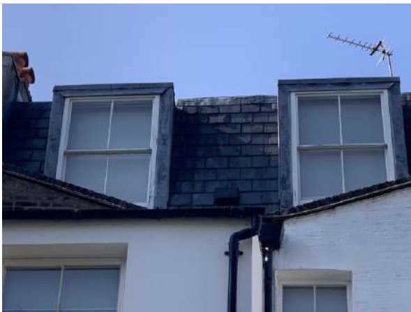
Photo 2 - Rear of main roof
