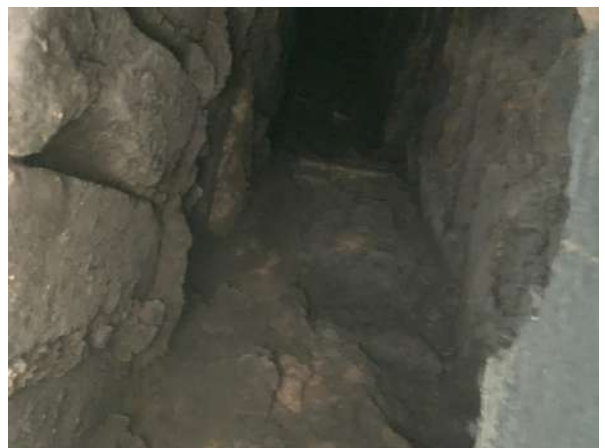
Photo 61 - Unlined flue
