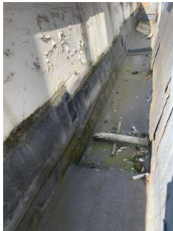
Photo 10 - Box gutter
