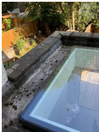
Photo 5 - Rear extension roof
