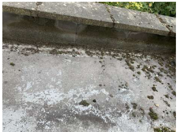
Photo 6 - Rear extension roof
