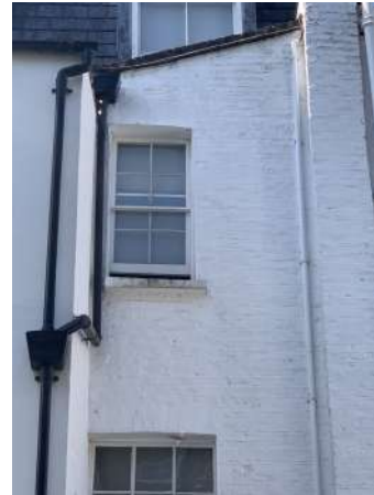
Photo 20 - Rear elevation main building
