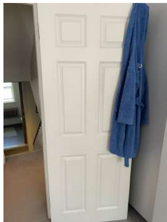
Photo 47 - Fire resisting door
